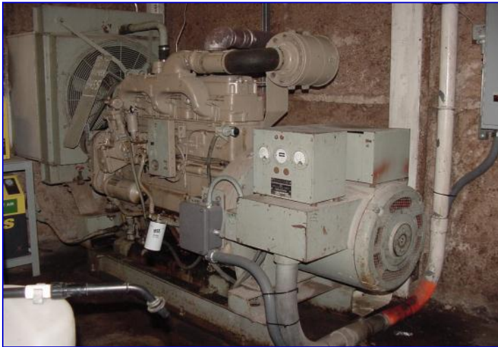
Emergency Diesel Generator
